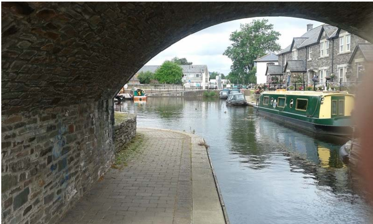
A view of Brecon Theatre Basin
