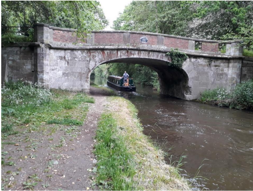
Teddesley Park Bridge or 'Fancy Bridge' in its day.
